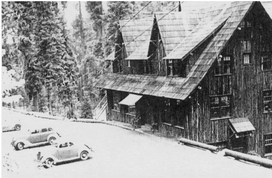
All buildings at Oregon Caves National Monument are sheathed in cedar bark, including the Chateau, seen here in this 1937 photo by Francis Lange.
